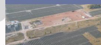
Western Downs Storage (2024 (1) )
